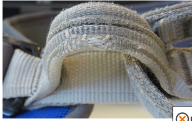
• Worn tie-in point
