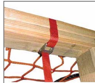
Cinch Straps installed on all four corners of the safety net.
