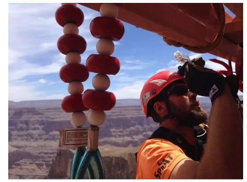
ClimbTech ANSI Z359 certified anchorage connector with sealed ball bearing rollers and spaces for ease while working on bridges or around pipe where other anchor points aren't prevalent.
